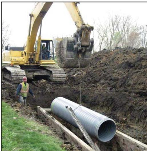
Photo illustrating sewer line installation.
